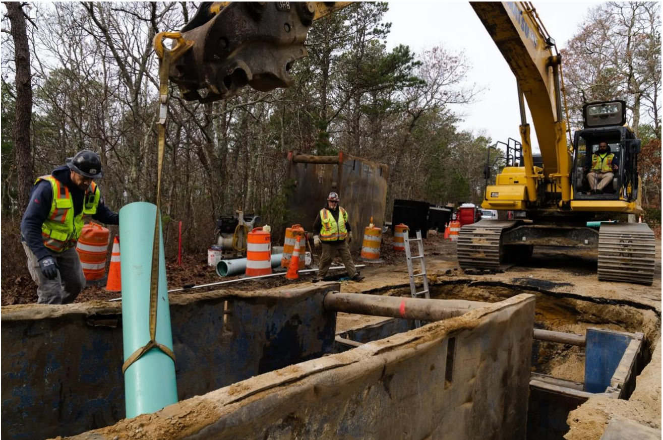
Workers installing a sewer line in Mashpee.
